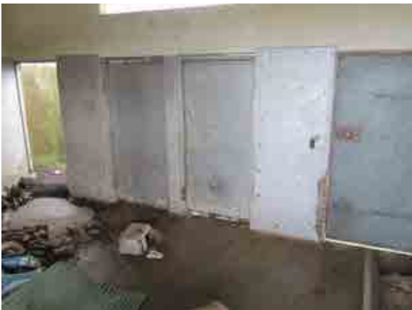
PICTURE 47 – VIEW OF THE STALL DOORS
