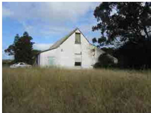
PICTURE 16 – THE NORTHERN FAÇADE
