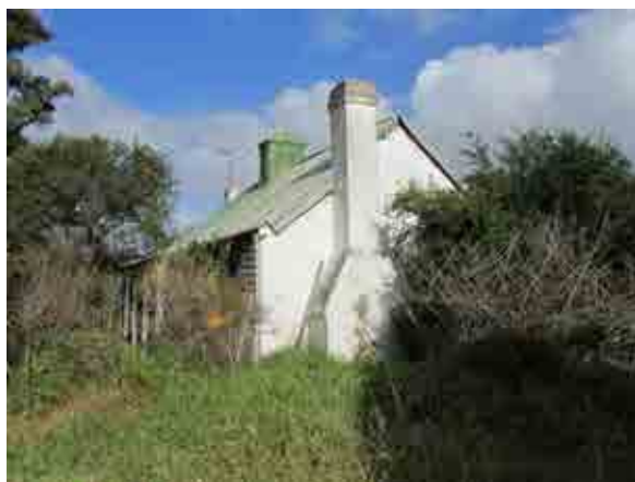
PICTURE 30 – THE NORTHERN MASONRY FAÇADE AND CHIMNEY
