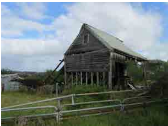
PICTURE 39 – VIEW SOUTHWEST TO THE TIMBER BARN
