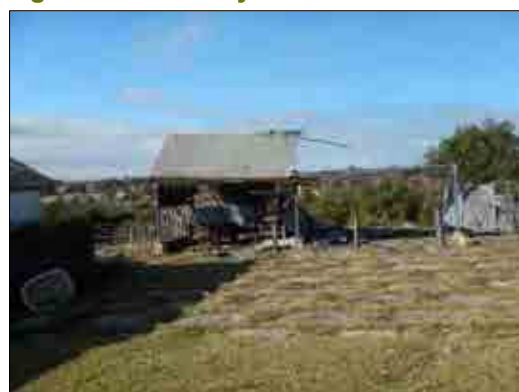
Figure 19: Westerly view of wool shed.
