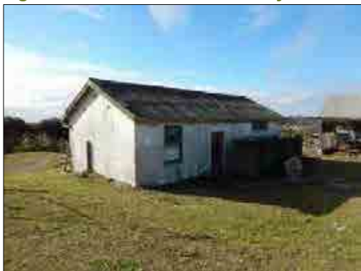
Figure 17: Rear view of the dairy.
