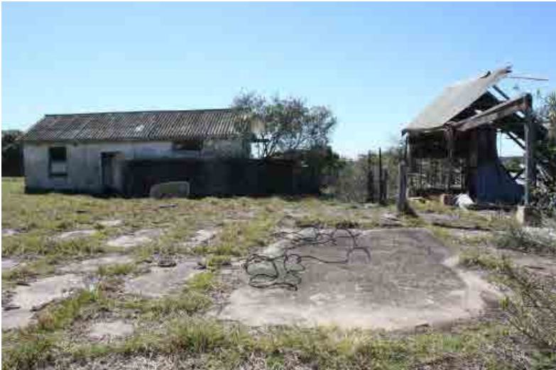
Figure 2.6 Rear of the Machinery Shed (4) with the collapsed timbers shed in area (6) to the right. Areas of concrete hardstand in the foreground may suggest an earlier shed that has now been removed.
