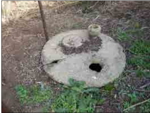
Figure 25: Well located adjacent to the slab hut.
