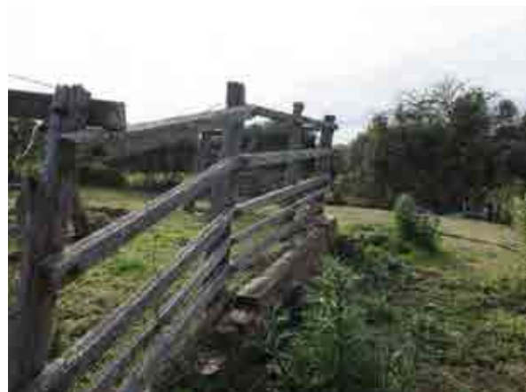
PICTURE 54 – LATER TIMBER FENCING
