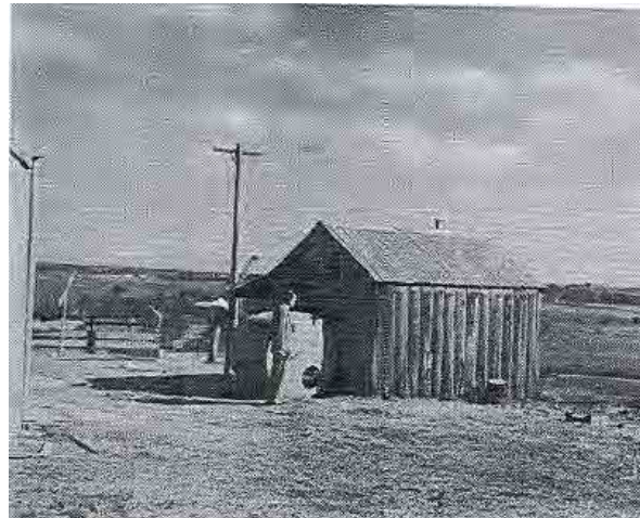
PICTURE 73 – THE TIMBER SLAB HUT (REAR VIEW)
