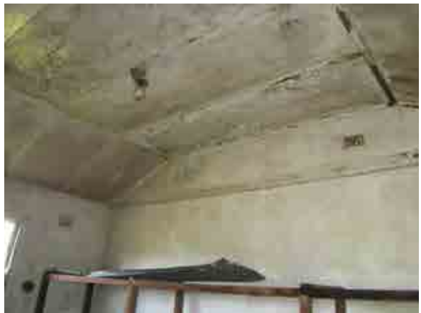
PICTURE 48 – VIEW OF THE VAULTED CEILING
