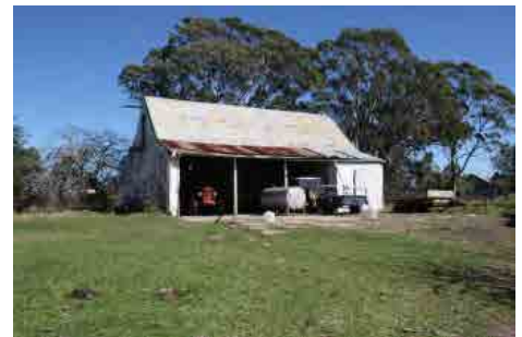
Figure 2.2 Eastern elevation of the Shingle roofed shed (1).
