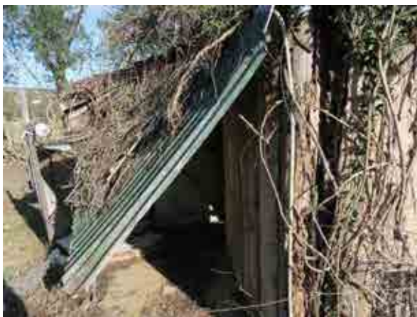
PICTURE 25 – VIEW TOWARDS THE SOUTHERN FAÇADE, SHOWING THE COLLAPSED VERANDAH ROOF
